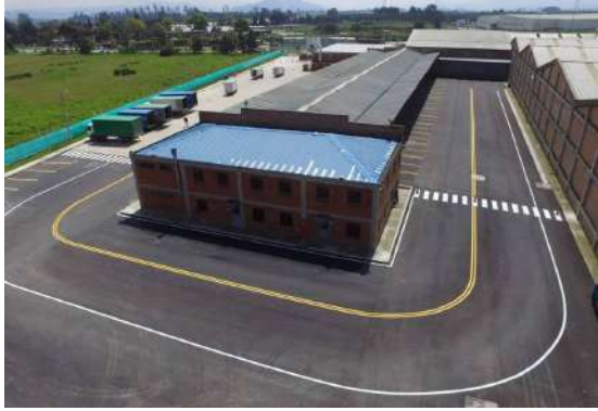
Adaptation of the Cayena Free Zone warehouse
