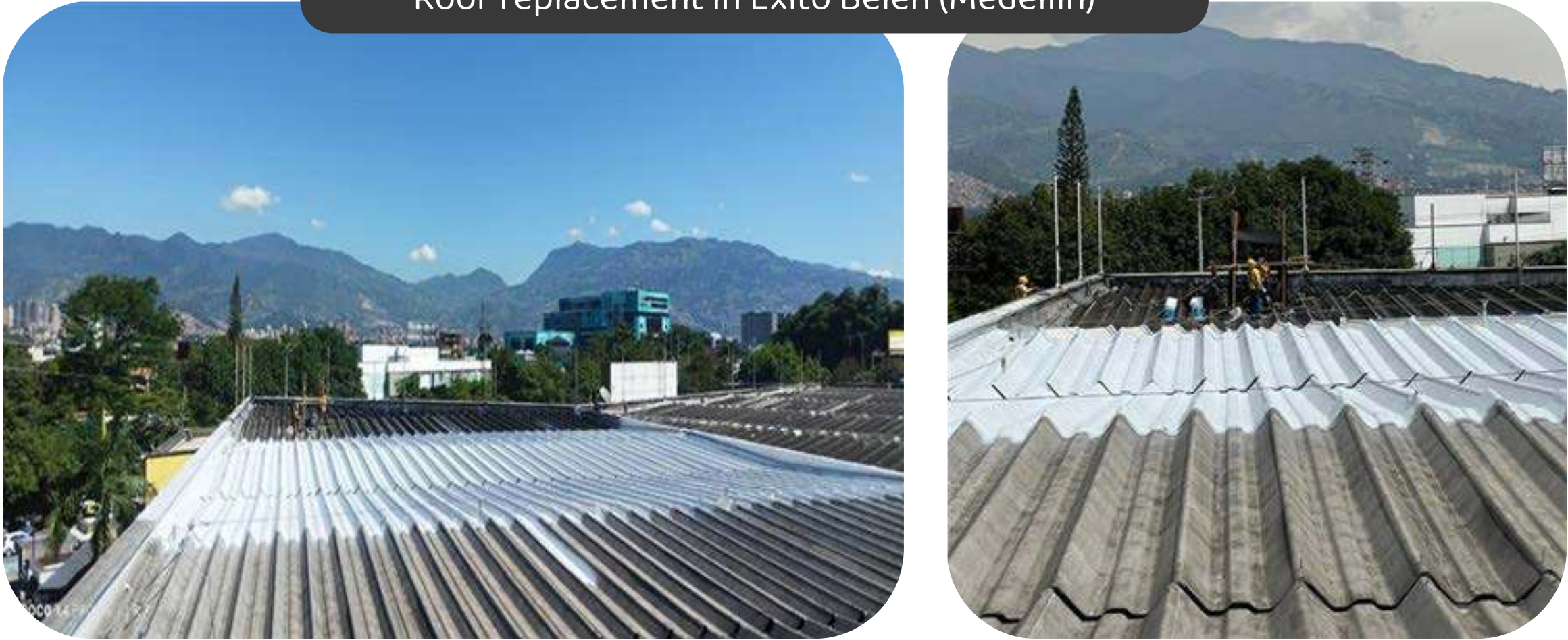
Roof replacement in Exito Belen (Medellin)
