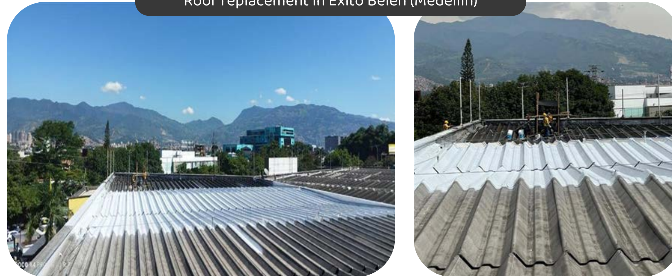
Roof replacement in Exito Belen (Medellin)
