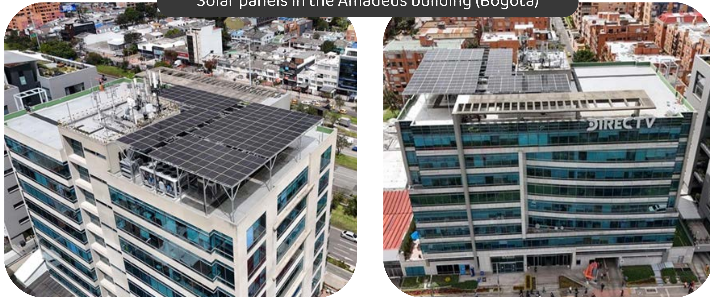
Solar panels in the Amadeus building (Bogota)
